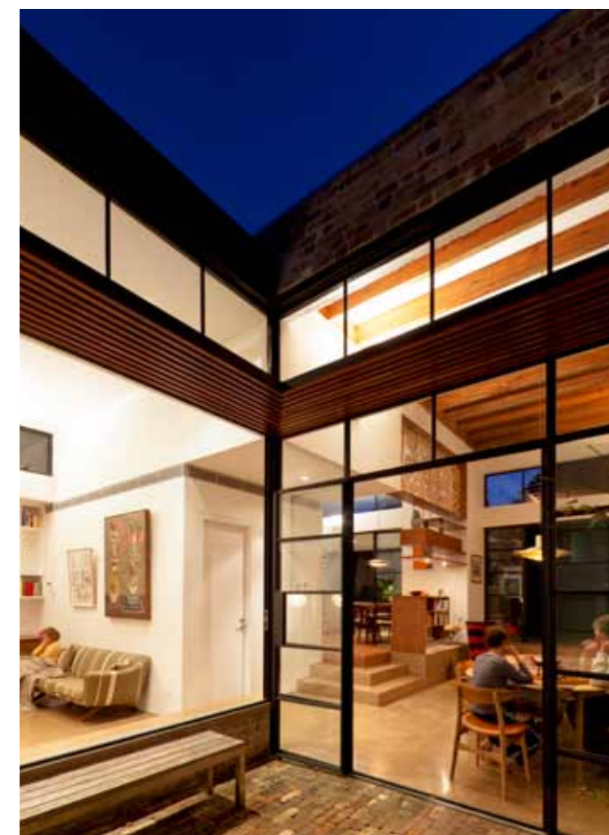
High windows capture year-round sunlight in this difficult orientation.
